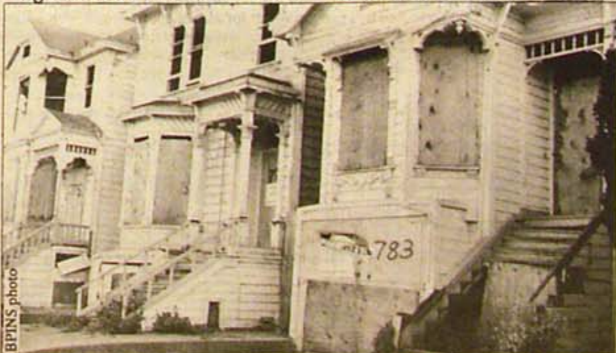
Oakland's Black and poor communities are full of abandoned houses due to redlining policies of city banks.
